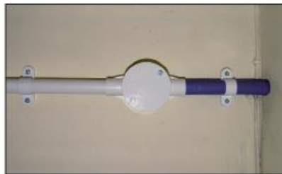
FIROBLOK CONDUIT SLEEVE FITTED INTO A 20MM BESA BOX
