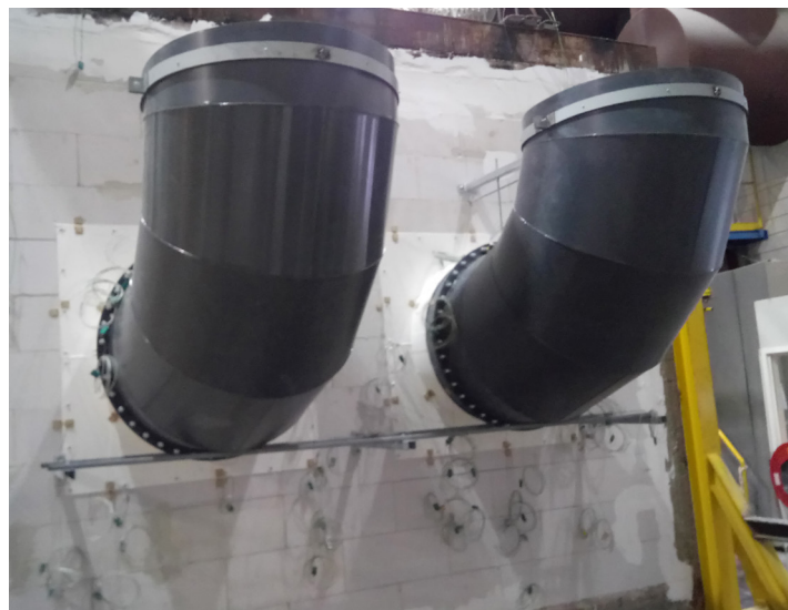
EXTERNAL VIEW BEFORE THE TEST BEGINS
